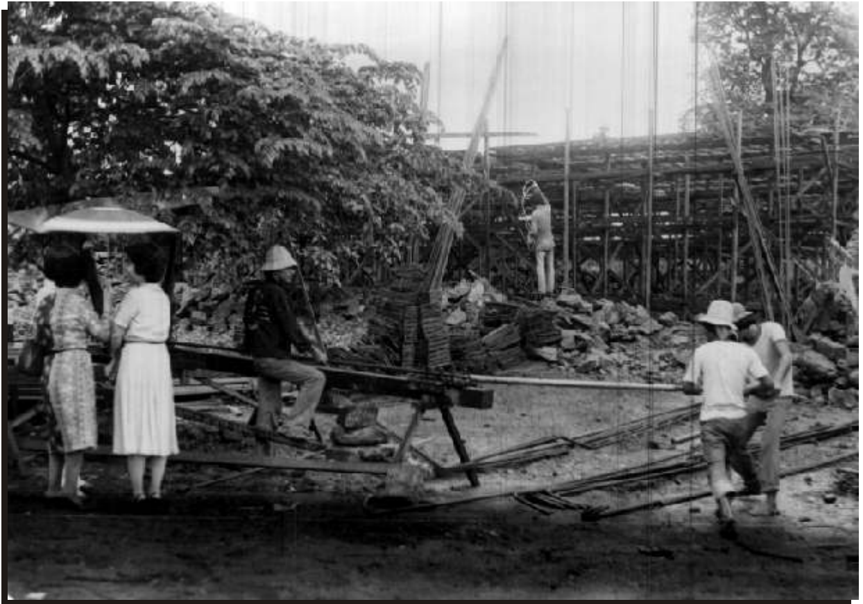
The PCS Building under construction in 1980
