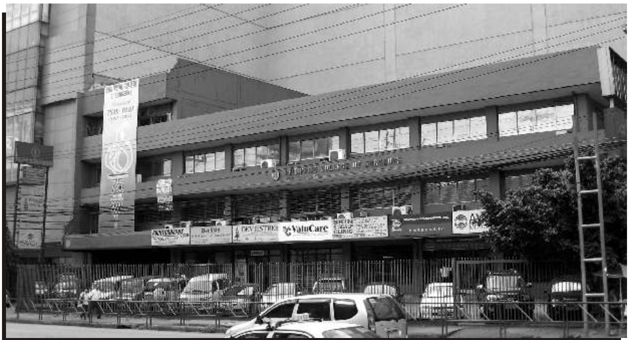
The PCS Building today
