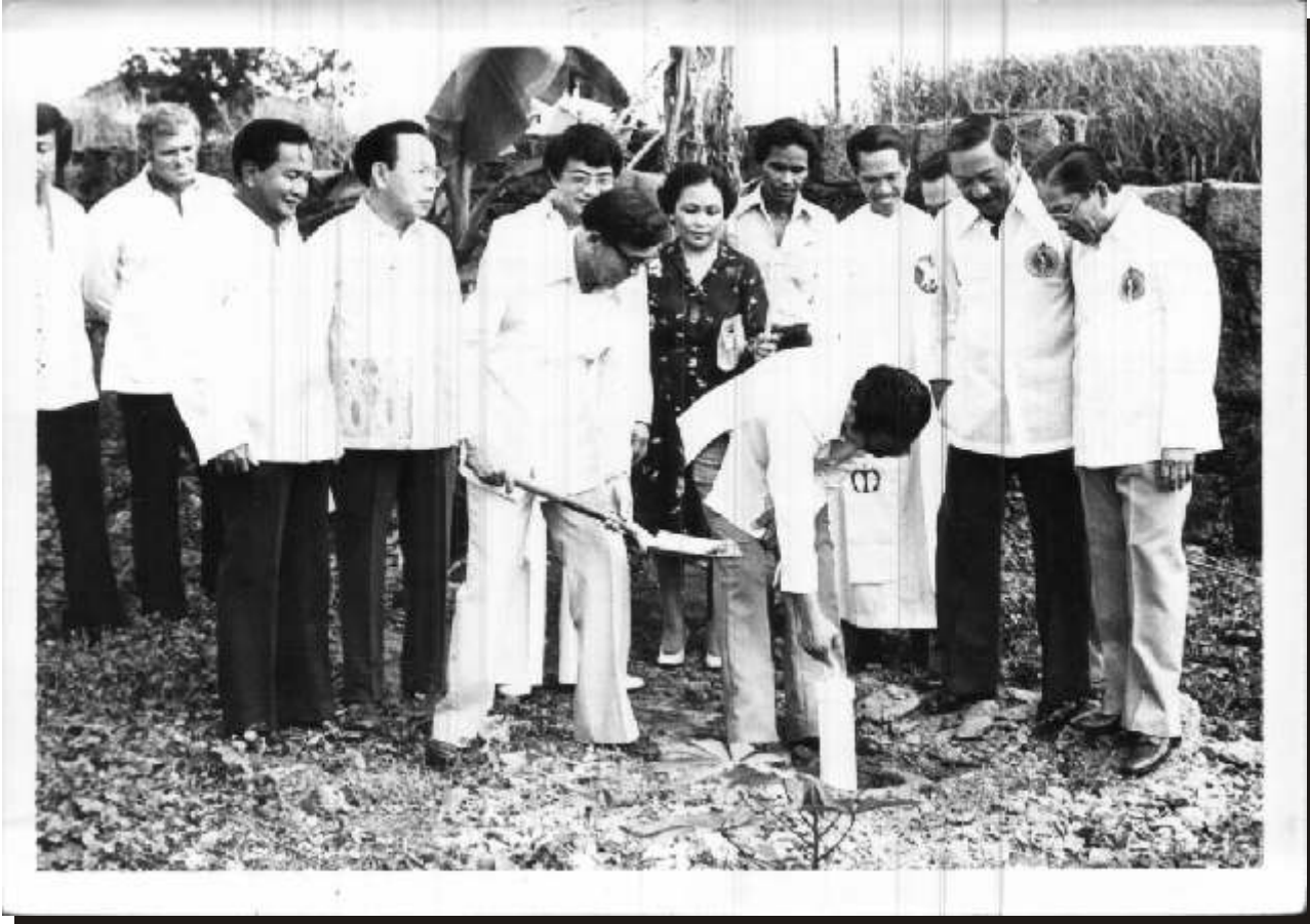
Cornerstone Laying Ceremony June 13, 1980 at the PCS lot along EDSA, Quezon City
